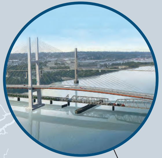
Pattullo Bridge Replacement Project
